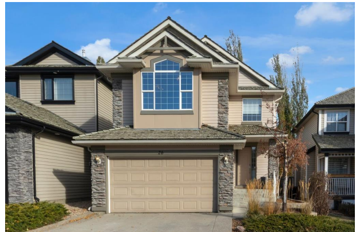
26 Springbank Rise SW, Calgary, AB
